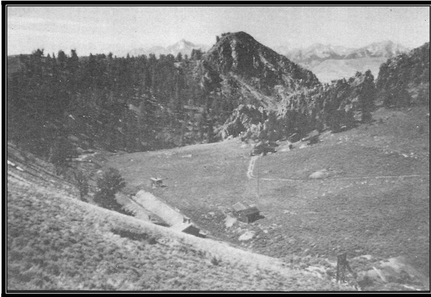
Figure 8. Camp buildings and mine dumps on the Nicholia Fraction. The rocks in the background are Kinnikinic Quartzite at the head of Cedar Canyon south of the Viola Mine (Anderson and Wagner, 1944, Plate 2A).
